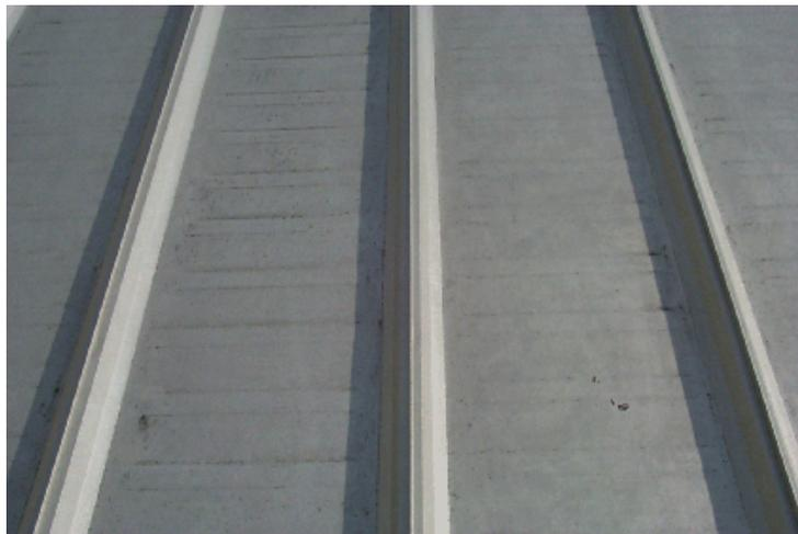
**Figure 5** Close-up of a typical acrylic coated 55% Al-Zn alloy coated sheet weathered roof
