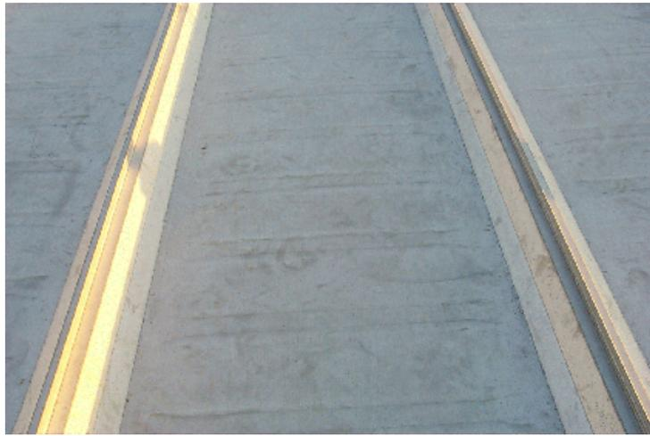
**Figure 5** Close-up of typical chemically treated 55% Al-Zn alloy coated sheet weathered roof
